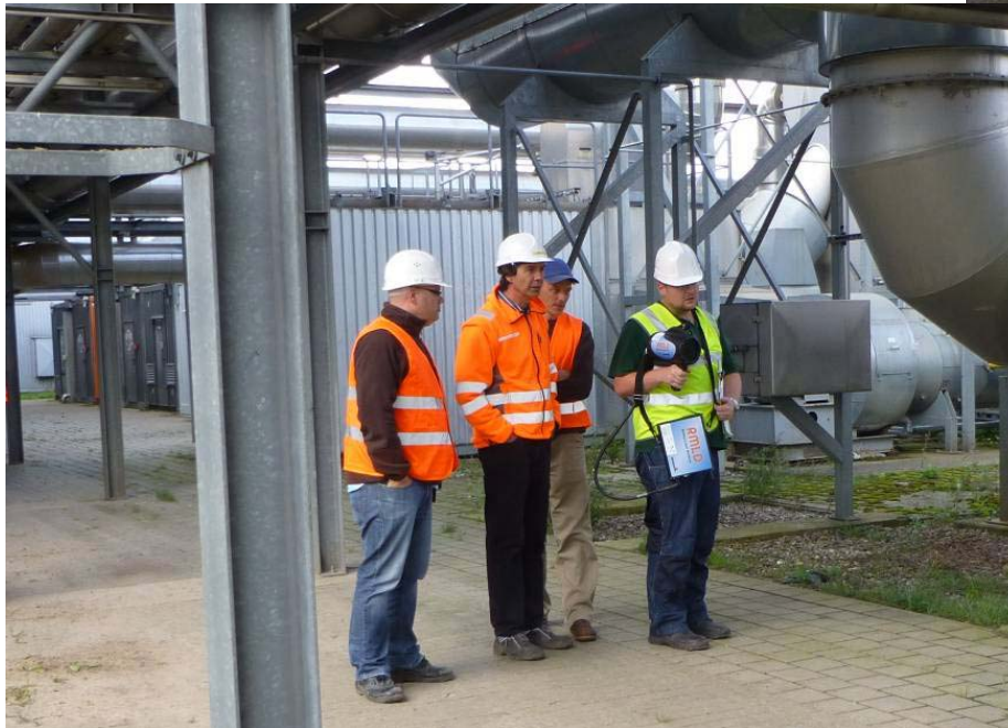
MBT / MBP– mechanical biologic pre-treatment plant
